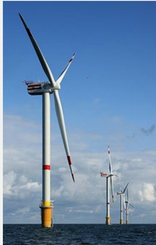
Wind turbines on the Belgian part of the North Sea. Source: © Hans Hillewaert
