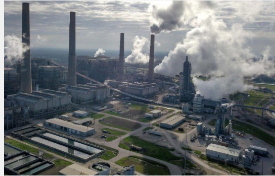
The structures in the right mid and lower are the carbon-capture column and related equipment at the Petra Nova facility.
